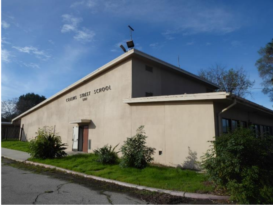
Figure 4. View looking southwest at the east and north façades of the Multi-Purpose Building. Source: ASM. February 9, 2017
