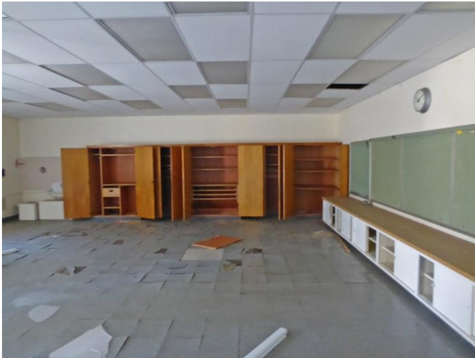
Figure 26. View of interior of Classroom Building A. Source: ASM. February 9, 2017
