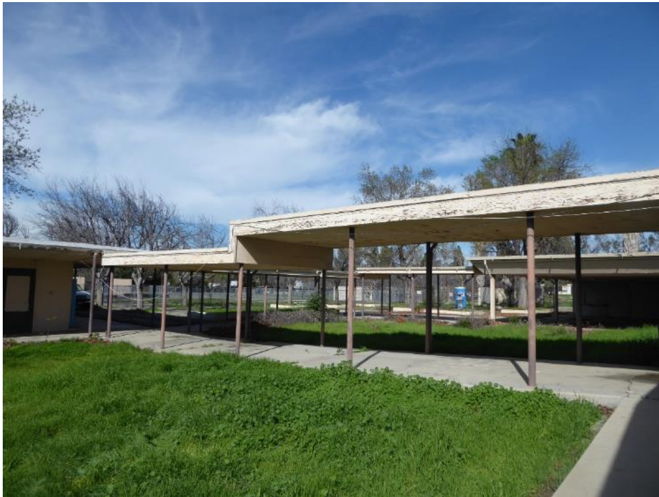
Figure 30. View looking southeast at the arcade system. Source: ASM. February 9, 2017
