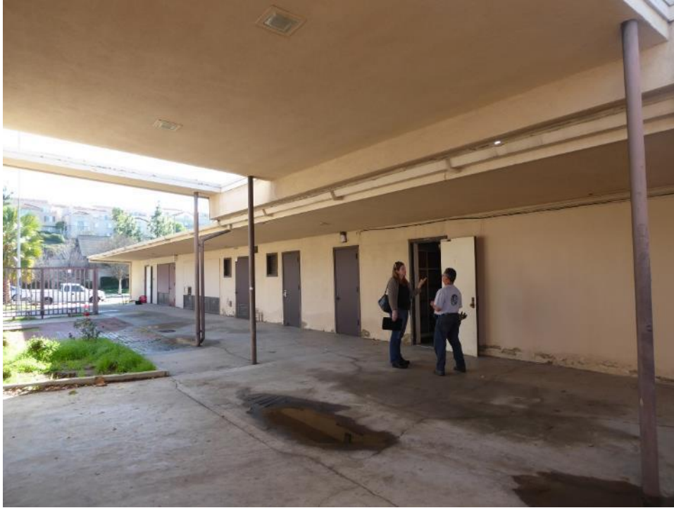
Figure 15. View looking southeast at the north façade of the Main Building. Source: ASM. February 9, 2017
