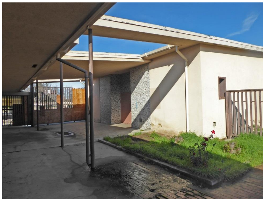
Image 3. View looking northwest at the main entrance to the school, with the Main Building on the left and the Multi-Purpose Building on the right. Source: ASM, February 9, 2017
