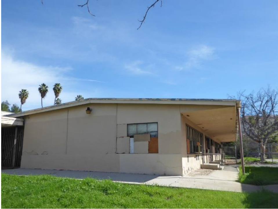
Figure 17. View looking northeast at the west and south façades of the Main Building. Source: ASM. February 9, 2017
