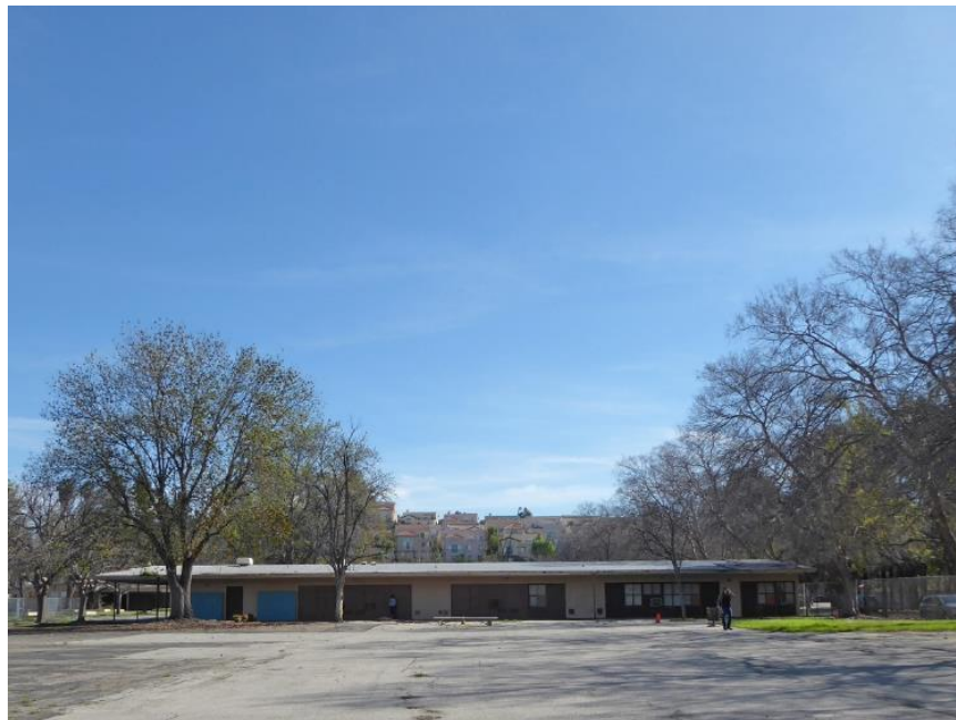
Image 1. View looking east at the west façade of Classroom Building B. Source: ASM, February 9, 2017
