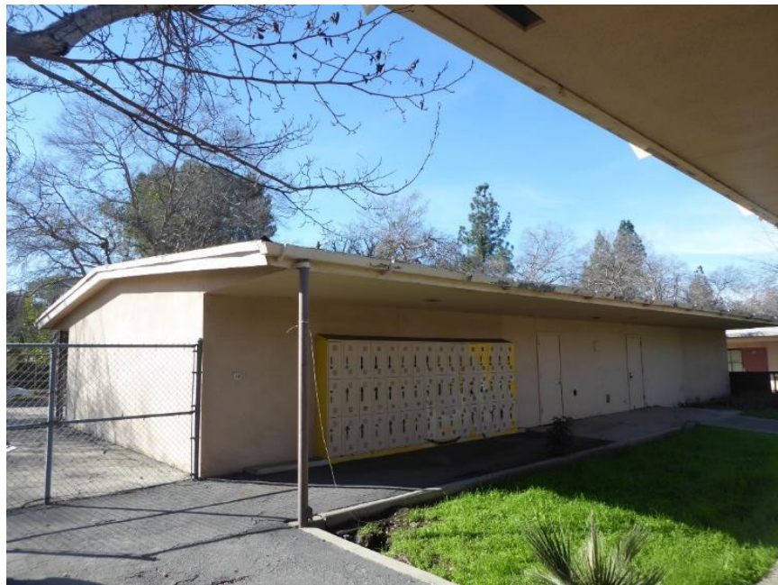
Image 1. View looking northeast at the west façade of Classroom Building A. Source: ASM, February 9, 2017
