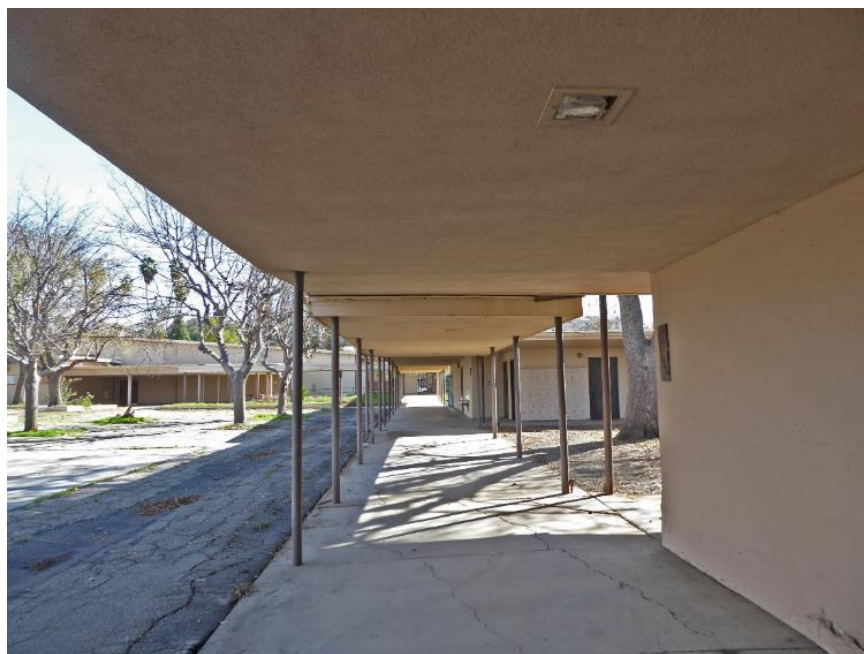
Image 2. View looking east at the central arcade. Source: ASM, February 9, 2017
