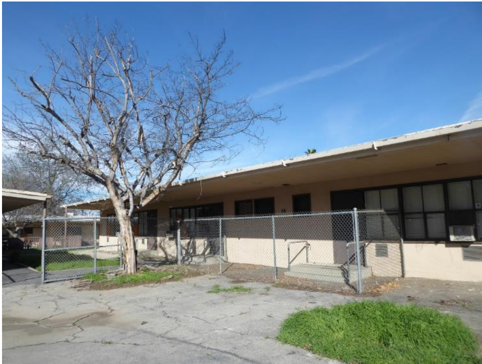
Figure 16. View looking northwest at the south façade of the Main Building. Source: ASM. February 9, 2017
