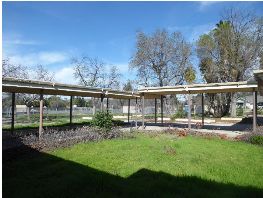
Image 3. View looking southeast at the arcade system. Source: ASM, February 9, 2017
