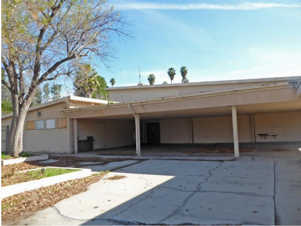
Figure 11. View looking northeast at the lunch pavilion, with the two wings of the Multi-Purpose Building to the rear. Source: ASM. February 9, 2017
