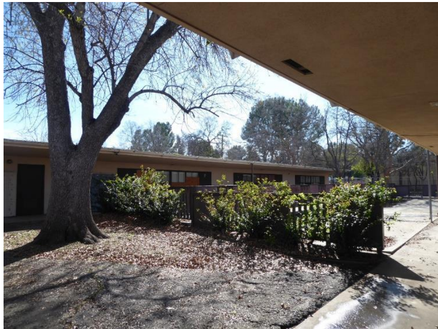
Image 2. View looking southeast at the west façade of Classroom Building A. Source: ASM, February 9, 2017
