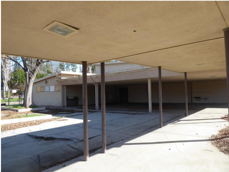
Figure 31. View looking northeast at the arcade system. Source: ASM. February 9, 2017
