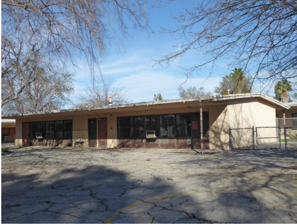
Figure 27. View looking northwest at the south and east façades of the Kindergarten Building. Source: ASM. February 9, 2017
