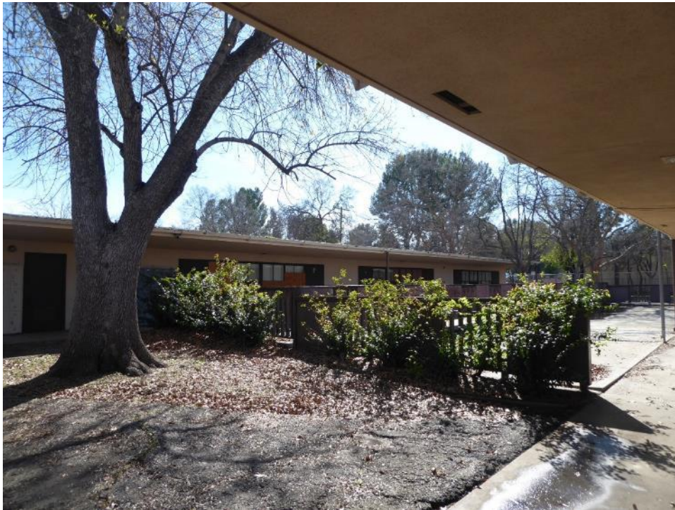
Figure 22. View looking southeast at the west façade of Classroom Building A. Source: ASM. February 9, 2017
