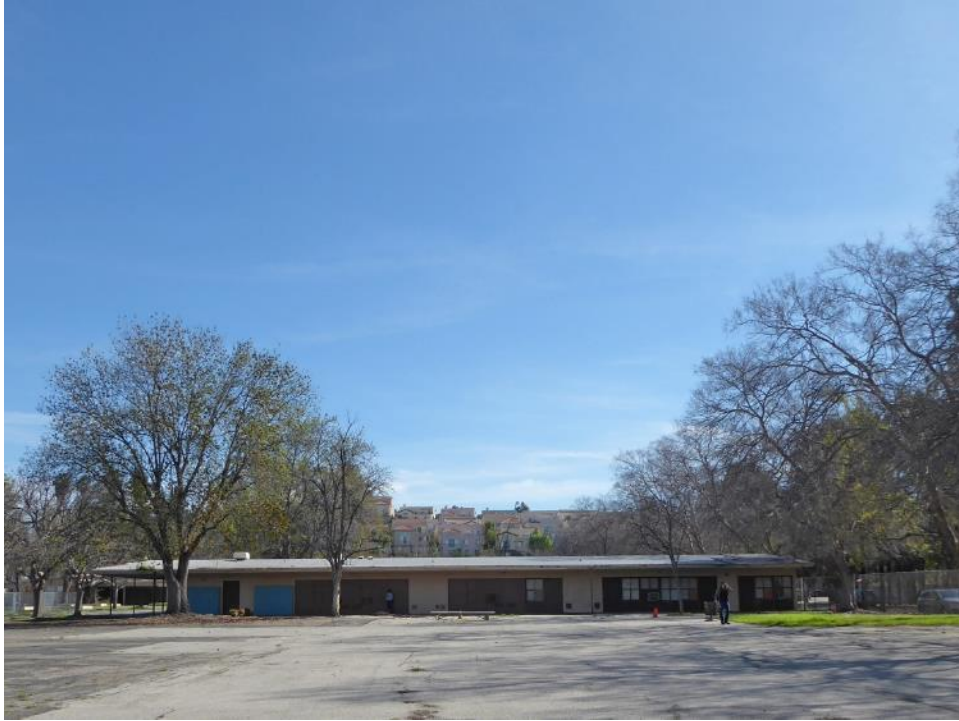
Figure 25. View looking east at the west façade of Classroom Building B. Source: ASM. February 9, 2017
