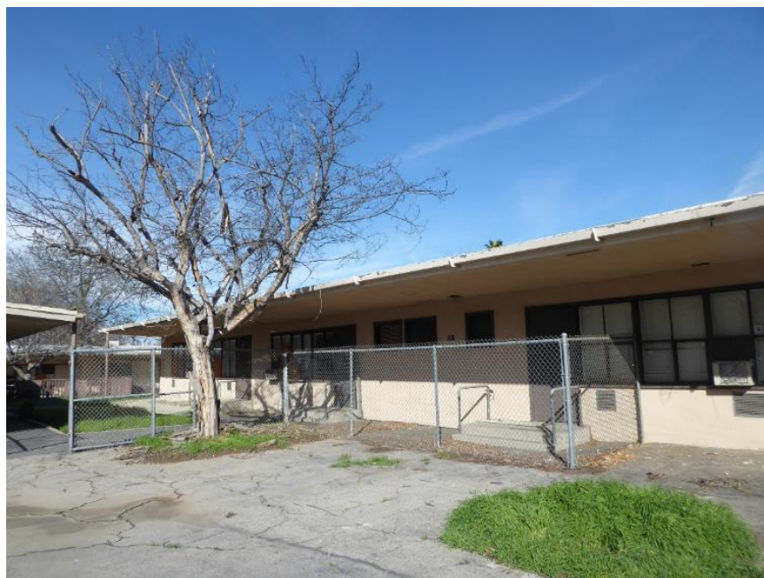
Image 3. View looking northwest at the south façade of the Main Building. Source: ASM, February 9, 2017
