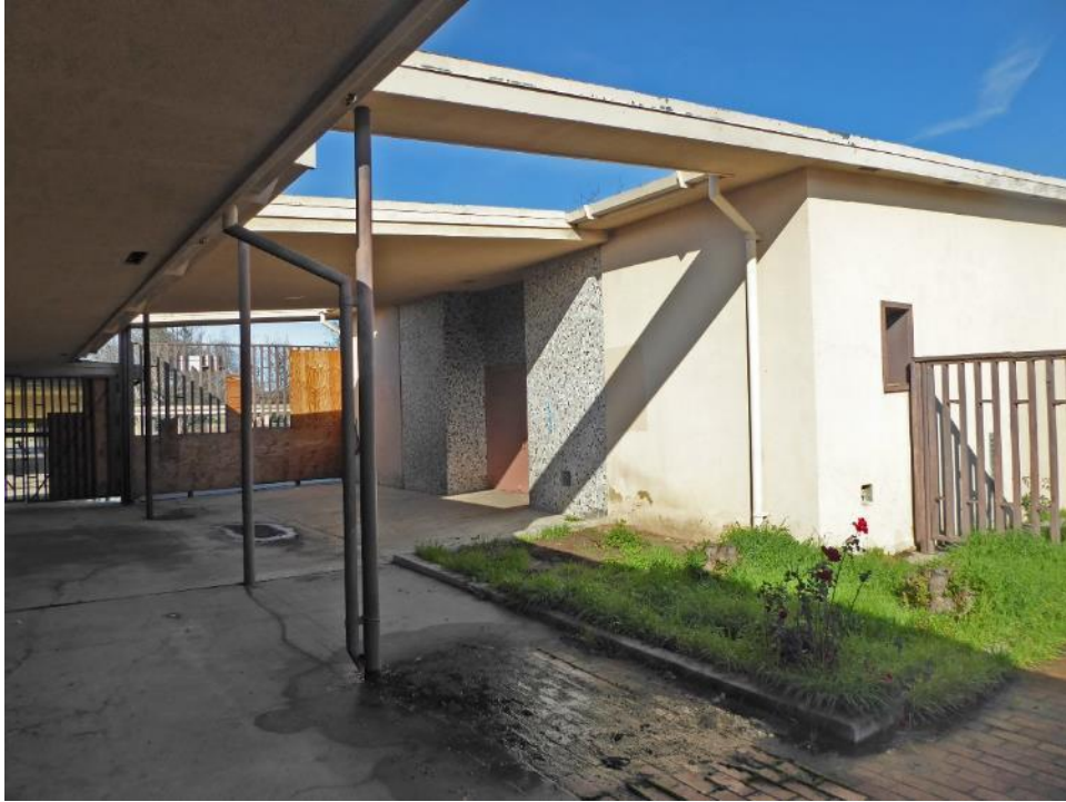
Figure 7. View looking northwest at the main entrance to the school, with the Main Building on the left and the Multi-Purpose Building on the right. Source: ASM. February 9, 2017
