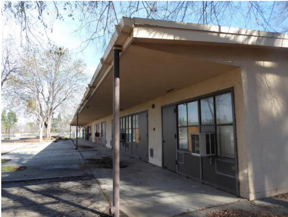
Figure 24. View looking northeast at the west façade of Classroom Building B. Source: ASM. February 9, 2017
