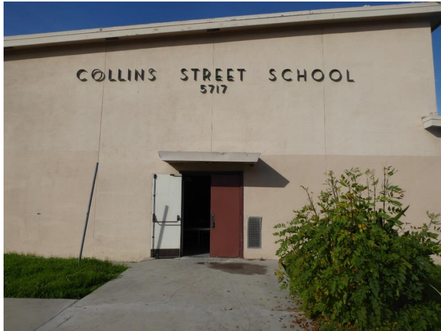
Image 1. Detail view of the entrance on the east façade of the Multi-Purpose Building. Source: ASM, February 9, 2017
