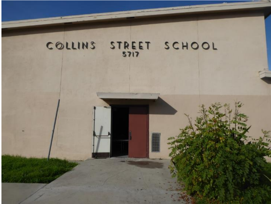
Figure 5. Detail view of the entrance on the east façade of the Multi-Purpose Building. Source: ASM. February 9, 2017
