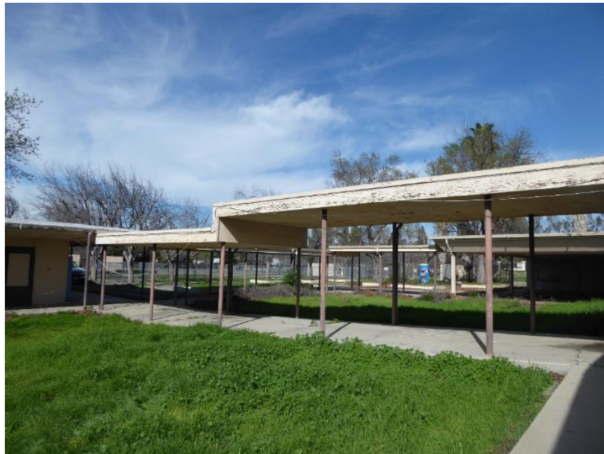
Image 1. View looking southeast at the arcade system. Source: ASM, February 9, 2017
