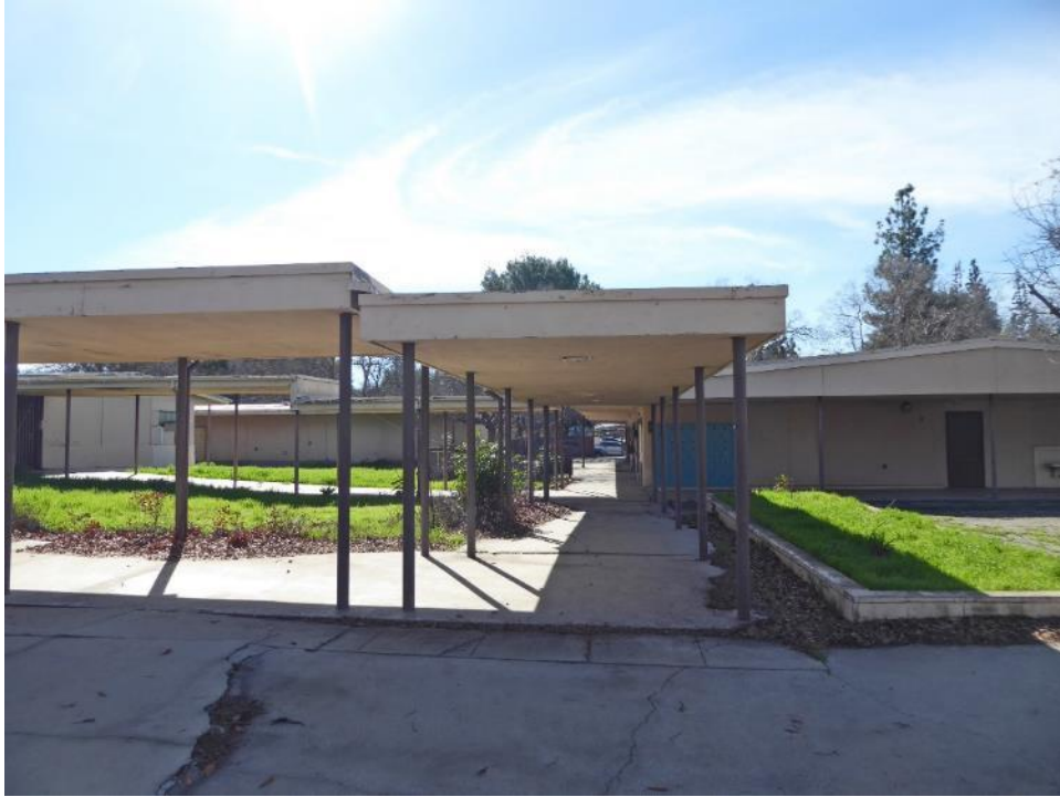
Figure 29. View looking south at the arcade system. Source: ASM. February 9, 2017
