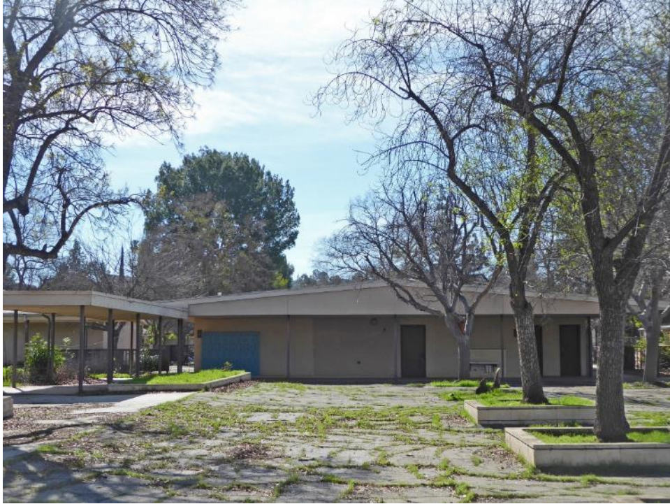
Figure 23. View looking south at the north façade of Classroom Building A. Source: ASM. February 9, 2017
