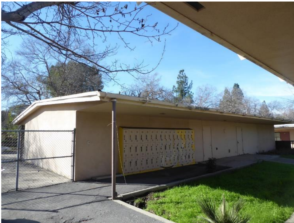
Figure 28. View looking southwest at the east and north façades of the Kindergarten Building. Source: ASM. February 9, 2017
