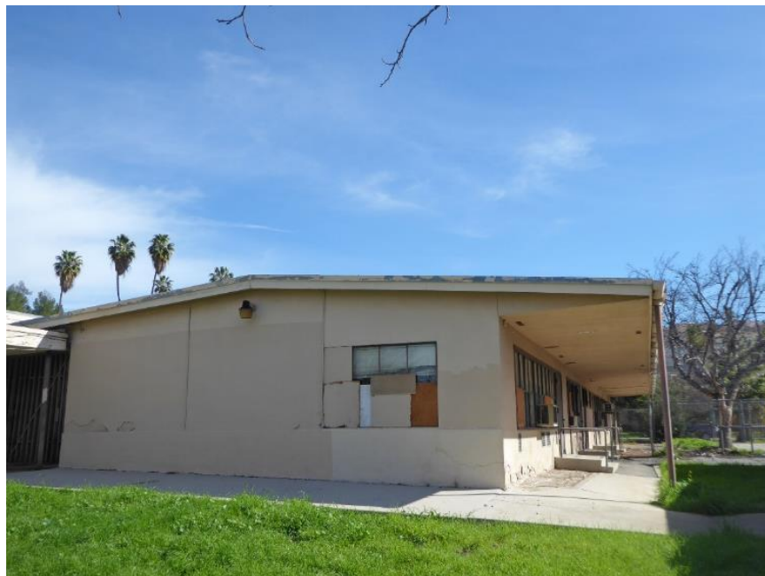
Image 4. View looking northeast at the west and south façades of the Main Building. Source: ASM. February 9, 2017
