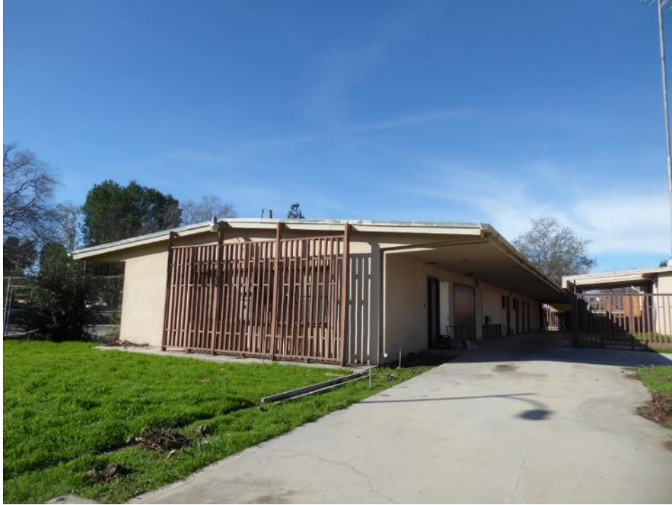
Figure 13. View looking west at the east façade of the Main Building. Source: ASM. February 9, 2017
